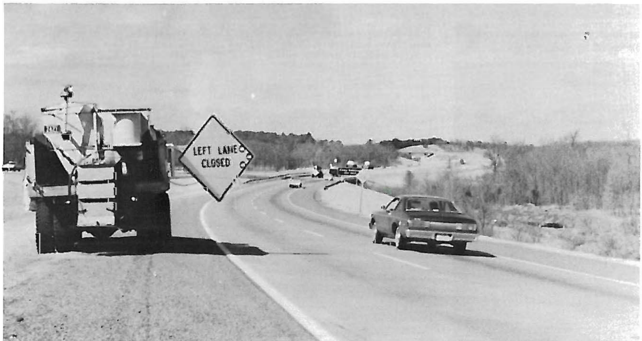
Signs mounted on trucks warn motorists of roadwork ahead. These types of signs are used in a moving or frequently moved type of operation.
