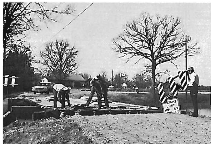
Highway and Transportation Department maintenance crews begin repairs to the State Highway 13 bridge near Humphrey.
