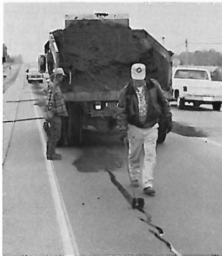
Joe Fedd, left, 1 year of service and Morris Bennett, 5 years service, both Single Axle Truck Drivers, seal cracks on roadway surface.
