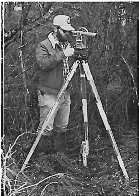
Mike Giles, Construction Aide with 8 years service, operates a transit to direct a line for a curve.
