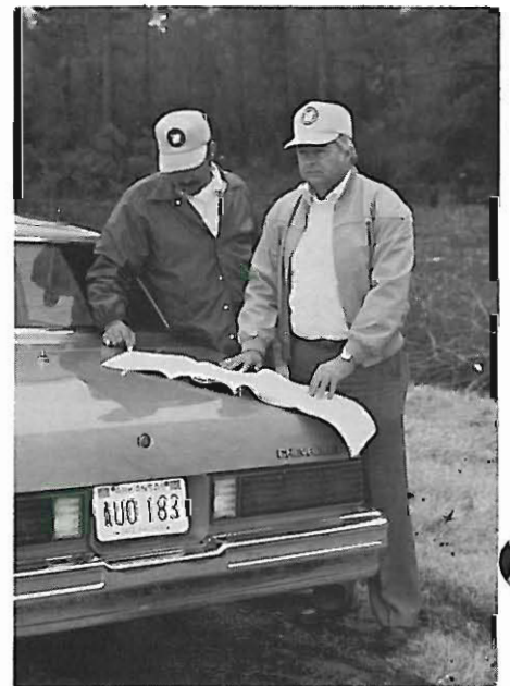
Texarkana Resident Engineer Ronnie Garner, left, with 16 years of service, and District Engineer Charles Mitchell, 22 years of service, review construction plans on the job site.
