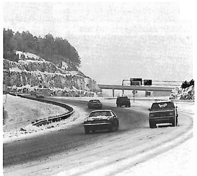
Interstate 430 at Highway 10 in Pulaski County.
