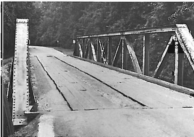
This one lane wooden structure is one of approximately 1800 deficient bridges on the Arkansas State Highway System in need of replacement. The department hopes to be able to replace 100 bridges each year.
